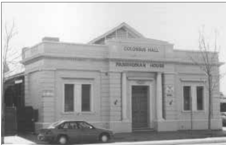
Colossus Hall, on Henley Beach Road, Torrensville.
