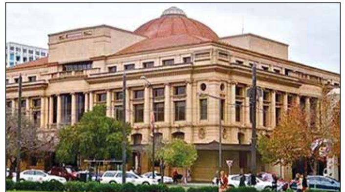
Sir Samuel Way Courts Building, Victoria Square
